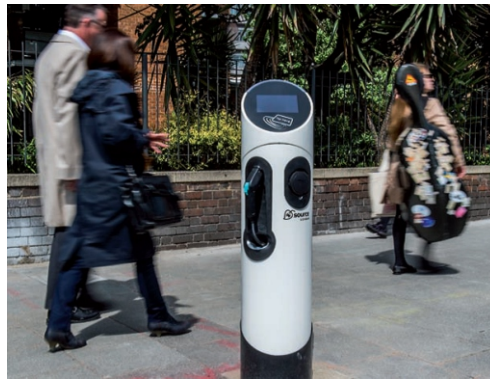
7kW charge point post
